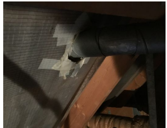
| Reparation af undertag
