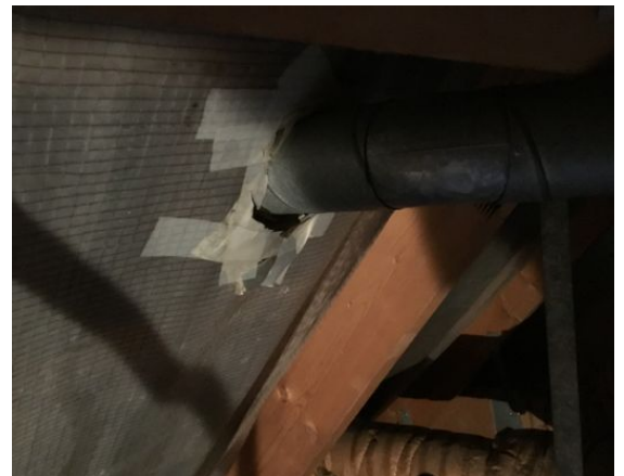
| Reparation af undertag
